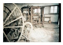
the cellar, the brick flooring here dates to the restoration. The floor had been lowered by about a foot at some point in time. There was a doorway on the south wall that was bricked over during the restoration because it was not original to the house. The well in the gift shop was probably used for cooling
